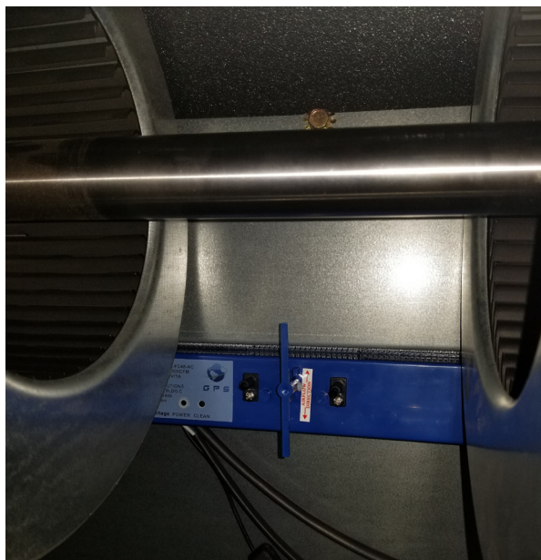
GPS-FC48-AC installed on a Unit Ventilator
